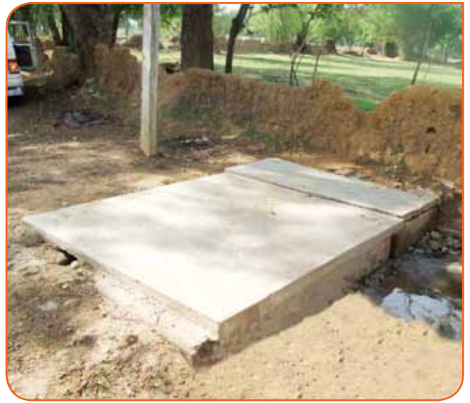
Water recharge pits at Chhotakitola village
