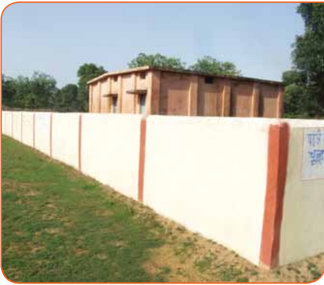
Boundary wall for a village school
