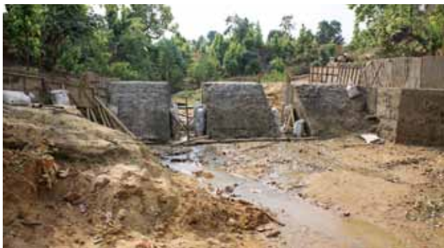
One of the stop dams constructed by us under the Water Shed programme
