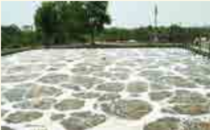
Additional aeration tank for effluent treatment
