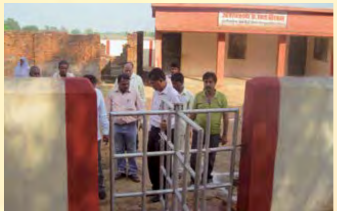
School boundary wall constructed under the Rajiv Gandhi Watershed Project
