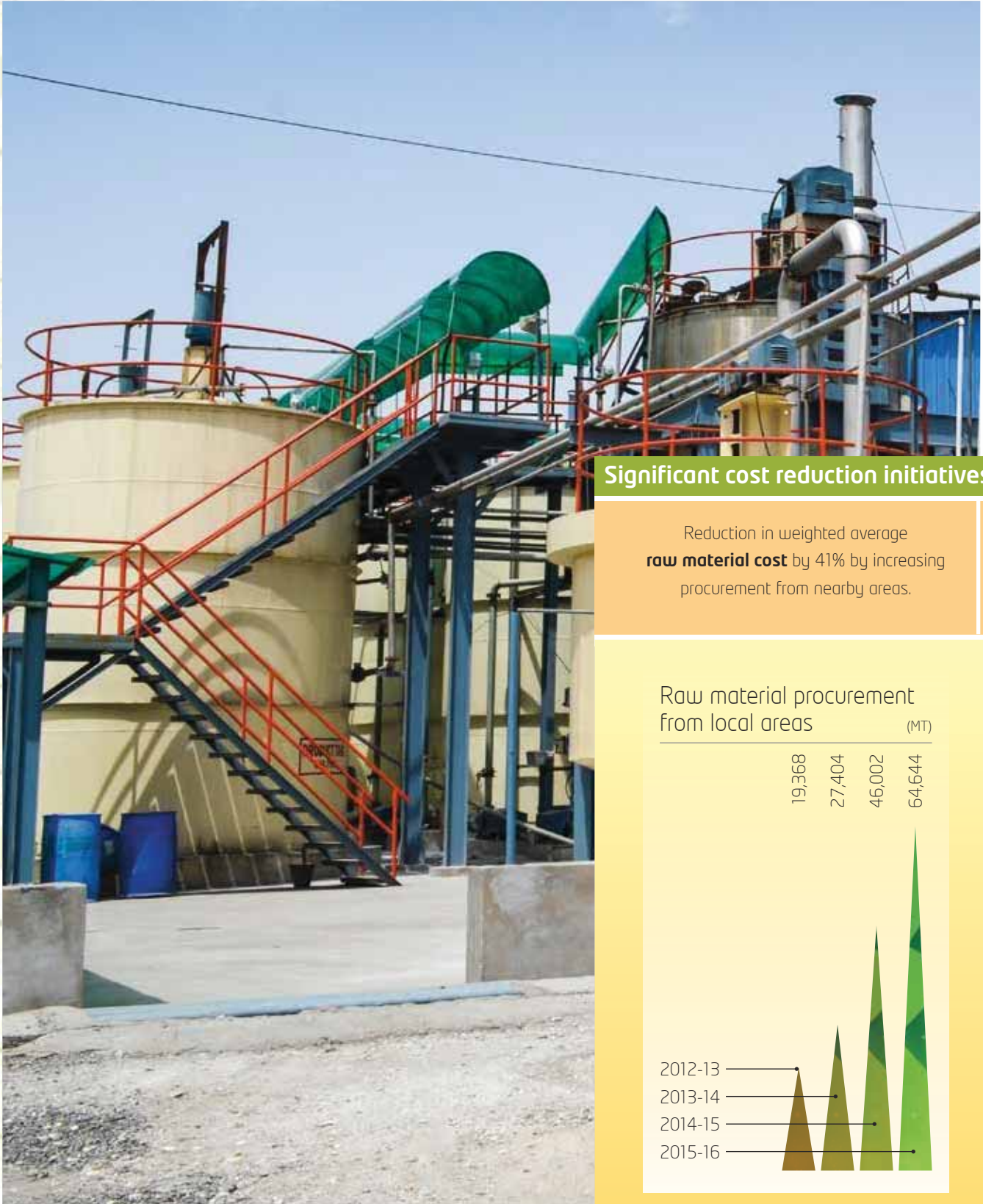
The new PCC plant
