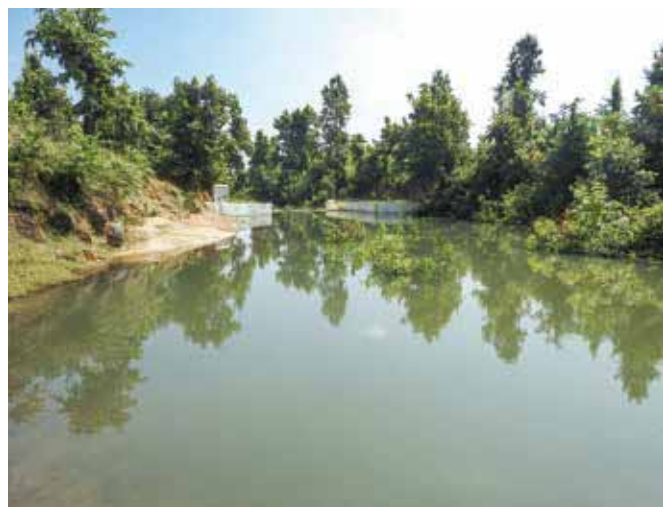
Stop Dam, Village Bhumkar
