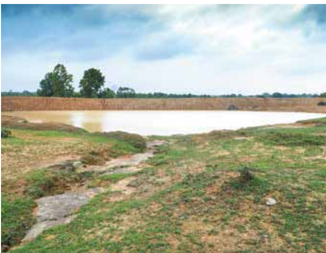
Earthen dam, Darshila
