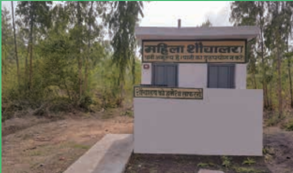
Female toilet built by Orient Paper
